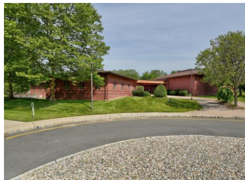
Montville Township Municipal Building
